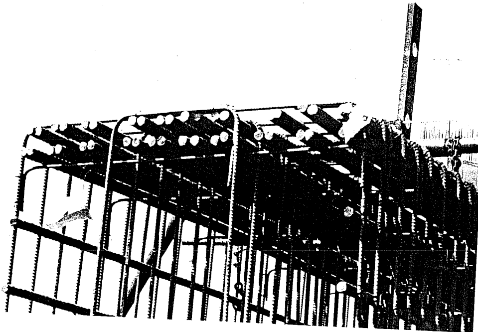
Figure 1.2 Reinforcement Cage
